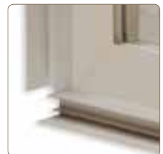
U-channel return accepts 3/4" and 1/2" material
